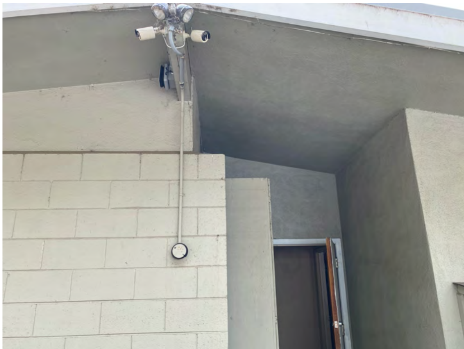
Photo 10- White Wood Fascia- 2515 Main St.- Exterior- Lead-Containing Paint (Good Condition)
