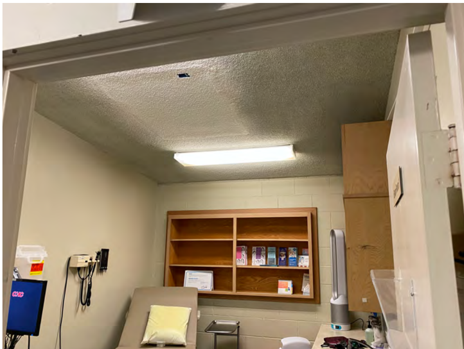
Photo 6- Spray-Applied Acoustic Ceiling Material- CHC Office Area- ACM
