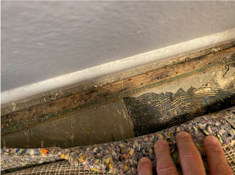
Photo 2- Gray 9" x 9" Floor Tile (Under Carpet & Sheet Flooring)- 2515 Main St.- CCHD Office Area- ACM
