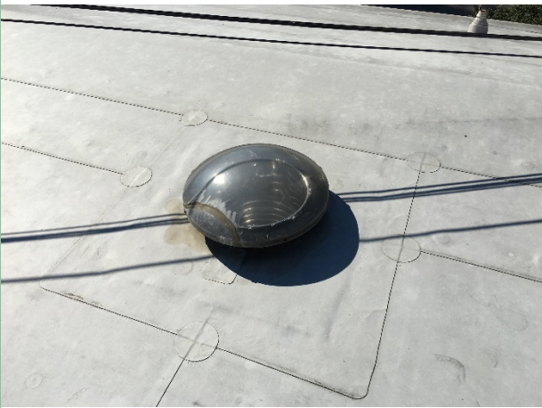
Roof with skylight
