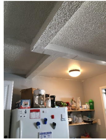
Ceiling at Kitchen
