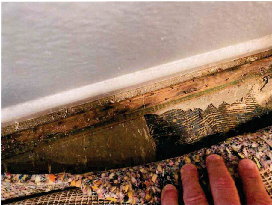
Photo 2- Gray 9" x 9" Floor Tile (Under Carpet & Sheet Flooring)- 2515 Main St.- CCHD Office Area- ACM
