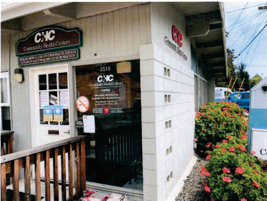
Photo 8- Gray Wood Window Casing/ Sill & Gray Wood Siding- 2515 Main St.- Exterior- LBP & Lead-Containing Paint(Poor Condition)
