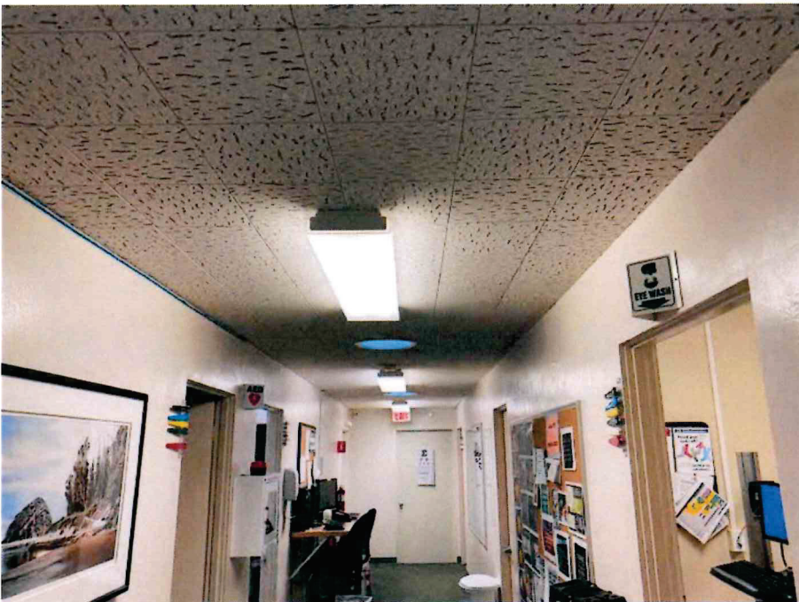
Photo 12- White Plaster Walls, White Wood Door & Casing- 2515 Main St.- CHC Area- Lead-Containing Paint & LBP (Good Condition)
