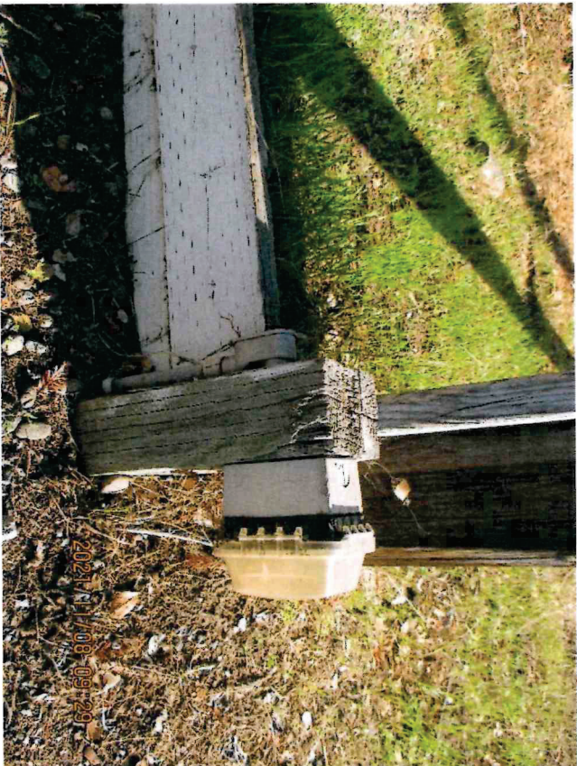
Photo 30. Non-compliant Exterior Convenience Outlet
