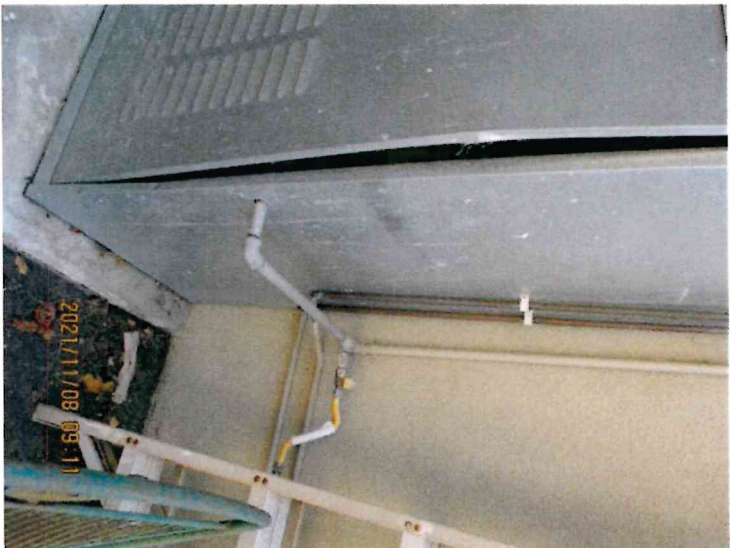
Photo 19. Non-compliant Gas connection
