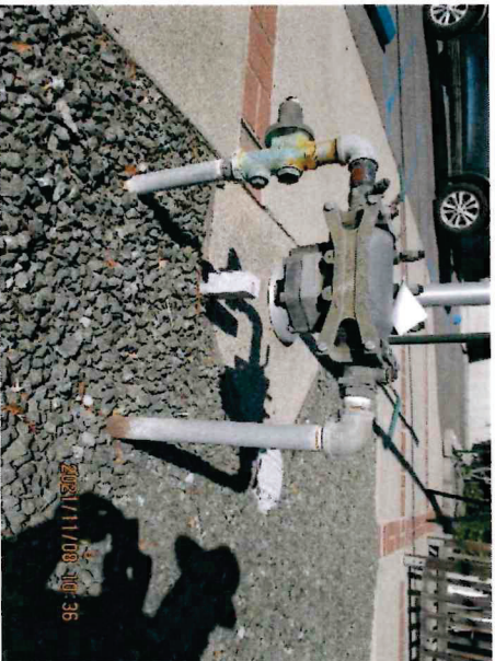
Photo 19. Non-compliant Gas connection
