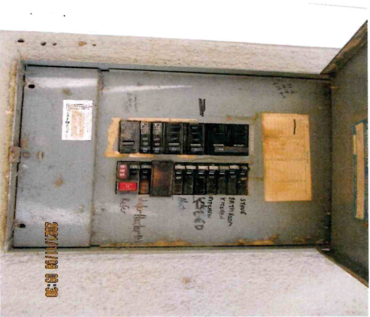
Photo 9. Wire Gutter Panel – Low Voltage Wiring View 10. Power Distribution Panelboard
